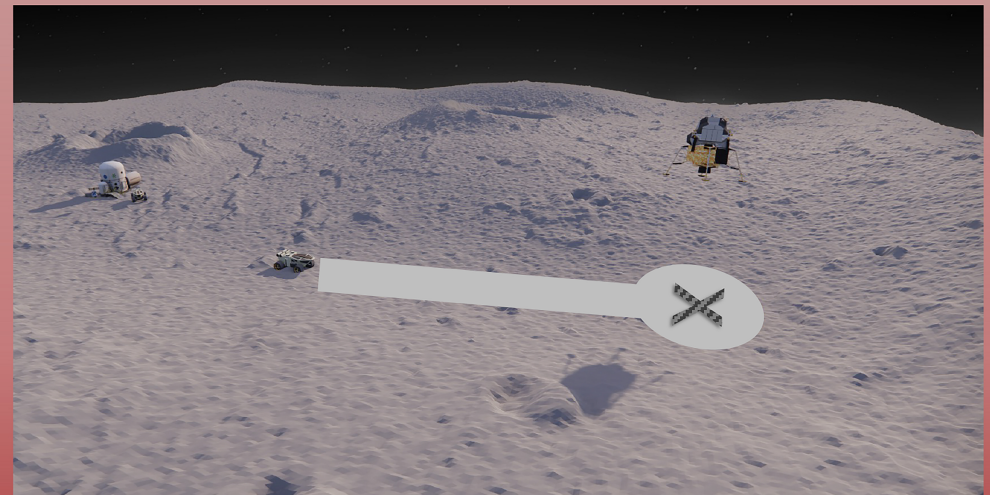
Figure 2: Rendering of cementitious Lunar landing pad with temporary roadway. Credit: Theo Wagner, Texas A&M University
